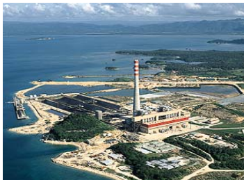
Pagbilao Power Station 2 X 367.5 MW
