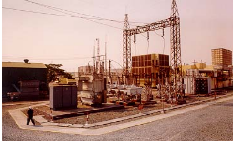
The Navotas Power Station
