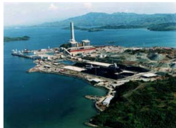
Sual Power Station 2 X 609 MW
