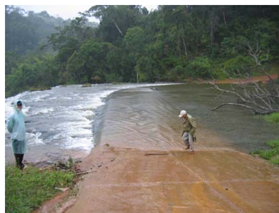
Krong Pa 2 waterfalls at intake site
